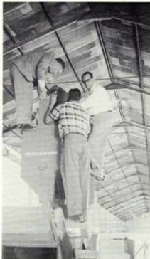
George Burditt looks over a 20" x 27" Wheelabrator Tumbler recently installed in the plant of Valvulas Rugo S.A. in Monterrey. In white shirt is Don Ruperto Gonzalez, Manager of plant. Man with plaid shirt is Ing. Rosendo Caballero.
